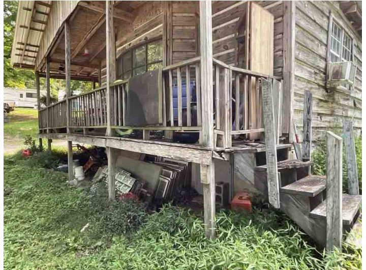
Damaged Deck
